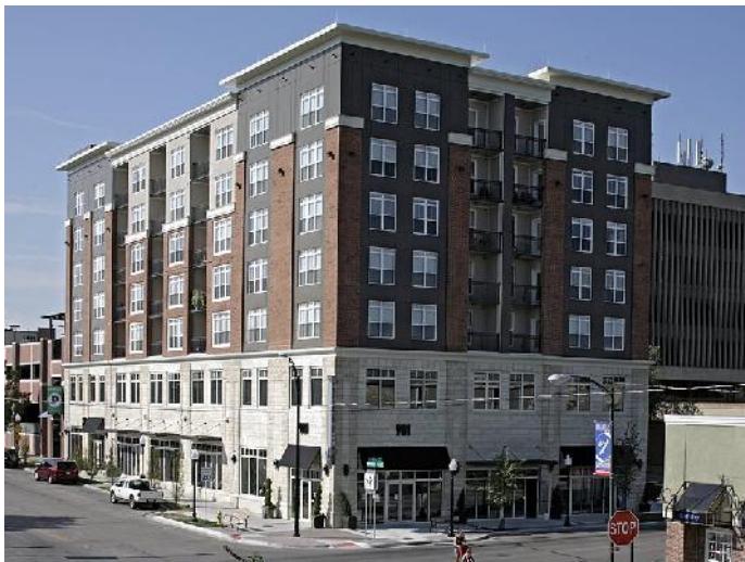
Upper story balconies are recessed along the façade, and a change of building materials and colors are used to break up the mass of the building.
