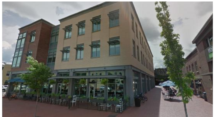
Example of incorporating bicycle facilities, a well-defined and compatible outdoor dining area, and off-street circulation.
