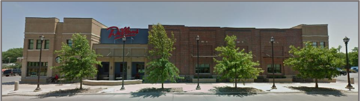
Example of new construction built at the property line with pedestrian oriented storefront elements, streetscape enhancements, well defined and modulating vertical building bays, and height deviations to create visual interest.
